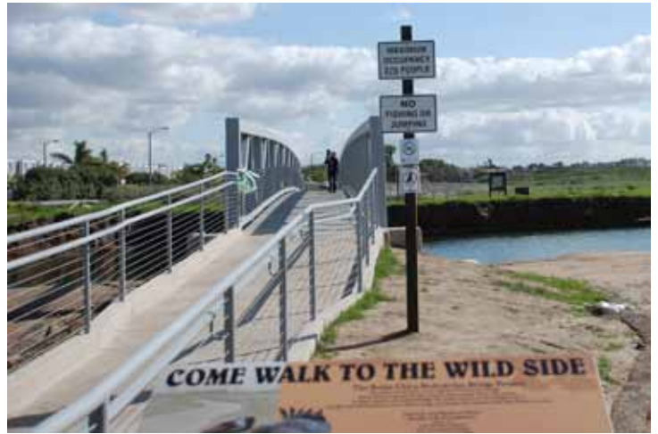
The new footbridge and signage near Warner Avenue.
